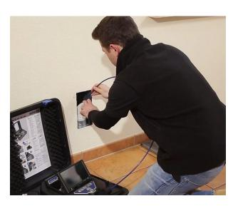
Watch our video on how to clean the Zehnder ComfoTube ductwork.
